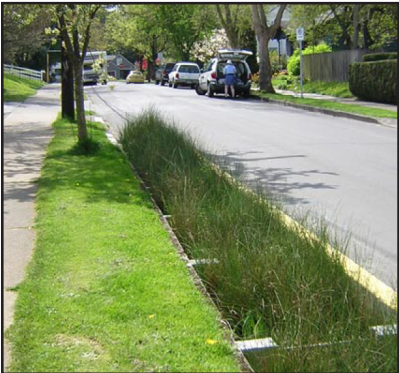
Figure 59: This green street retrofit is designed with a narrow curb extension that captures runoff from an existing crowned street.
