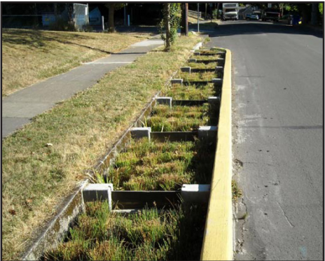
Figure 58: An example of a stormwater curb extension that reduced project costs by leaving the existing street curb in place.
