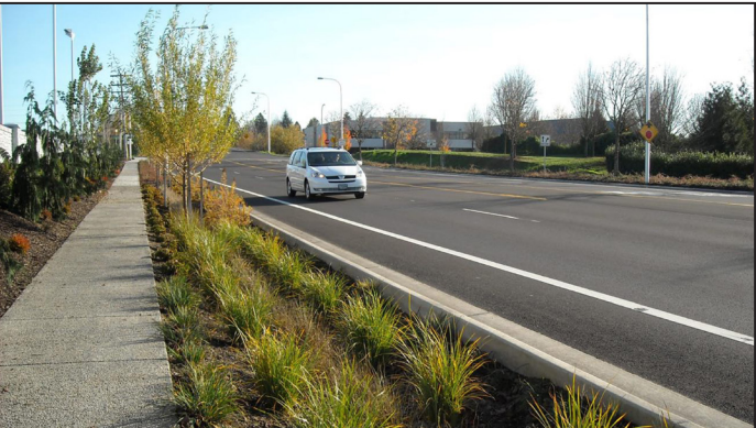
Figure 57: This arterial street utilizes a vegetated swale to accept stormwater from the street. This green street also uses sidewalks made from pervious concrete.
