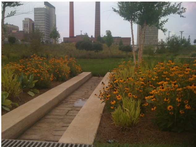
Figure 66: Biofiltration System at Railroad Park
