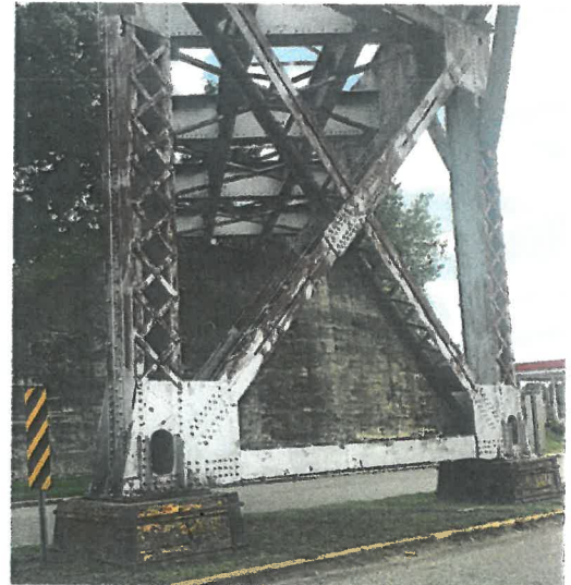
Example of abandoned railroad infrastructure.
