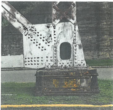
Abandoned railroad infrastructure, detail.
